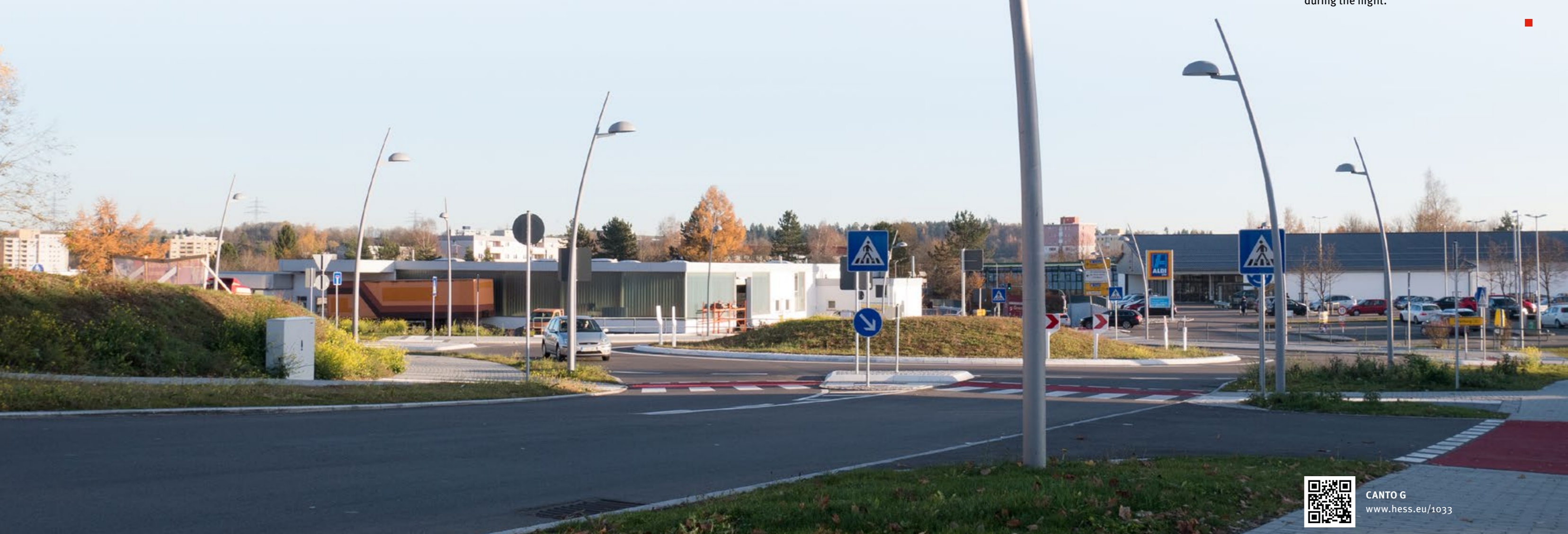
The new roundabout at the junction Milanstraße / Vorderer Eckweg ensures a smooth traffic flow into the industrial area.
